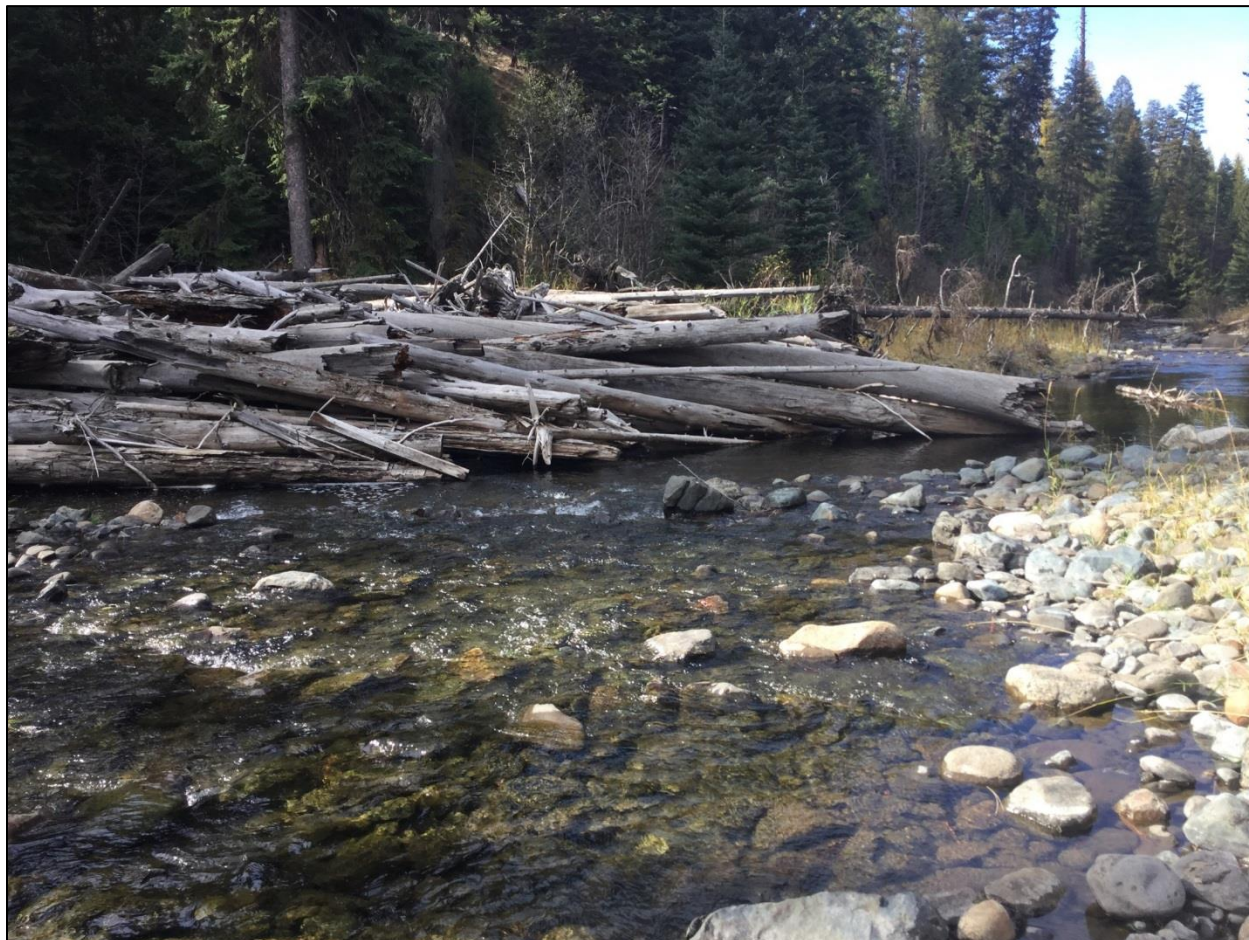
Figure 3-5. Example Natural Log Jam near Station 110+00
